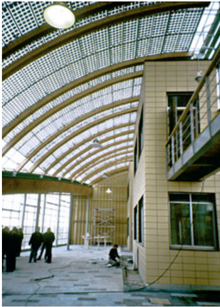
Fig.1 This curved roof of a commercial building conservatory space in the Netherlands is formed by PV modules [2]. Such curved PV surfaces limit string connection options.
