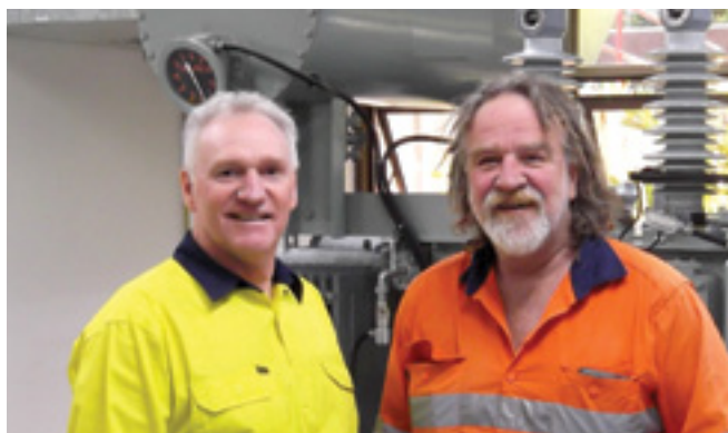
Both Platinum Members, Kerry Williams (K-BLK Power) with Jon Ford (Maxivar) at the final commissioning of the transformer in July.
